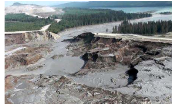
Mt. Polley Dam Failure
